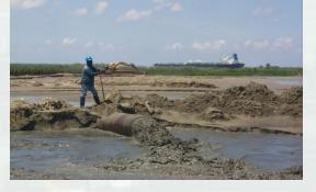
Spreader plate for hydraulic pipeline discharge
