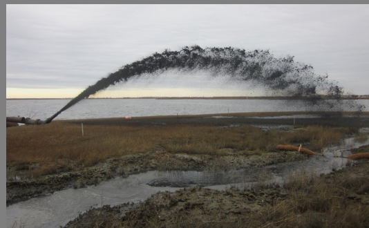
Thin layer sediment placement site at Avalon Marsh to restore shoreline edge and fill pannes. Photo taken from NJDEP Office of Dredging and Sediment Technology (Pecchioli 2015).
