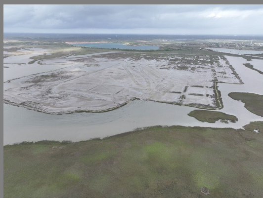
Thin layer sediment placement site at Pierce Marsh Preserve to restore 115 acres of marsh habitat. Photo taken from NOAA Guld Spill restoration.
